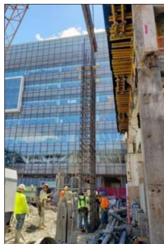
Cage Splice "Over the Hole"
