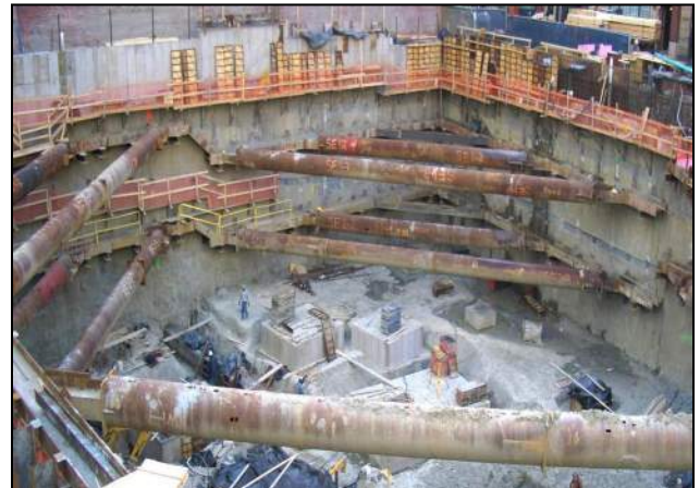
Braced Slurry Wall
