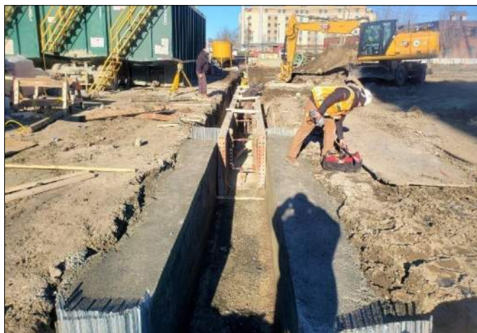
Guide Wall Construction
