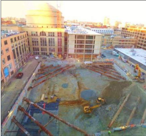
Slurry Wall Near Existing Buildings
