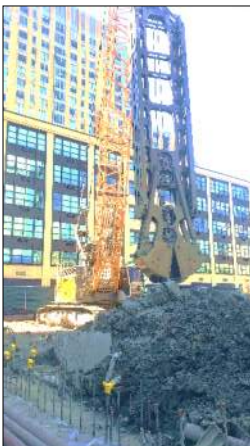
Various Obstructions Encountered During Slurry Wall Excavation
