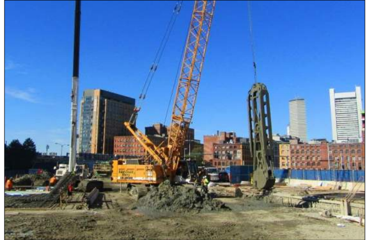
Slurry Wall Excavation
