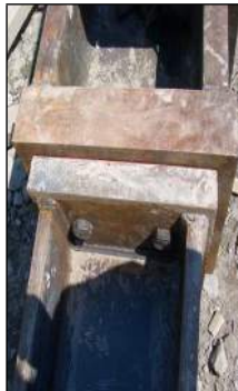
Lifting Head Splice
