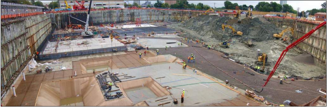
Completed Slurry Wall Acting As Temporary Earth Support System
