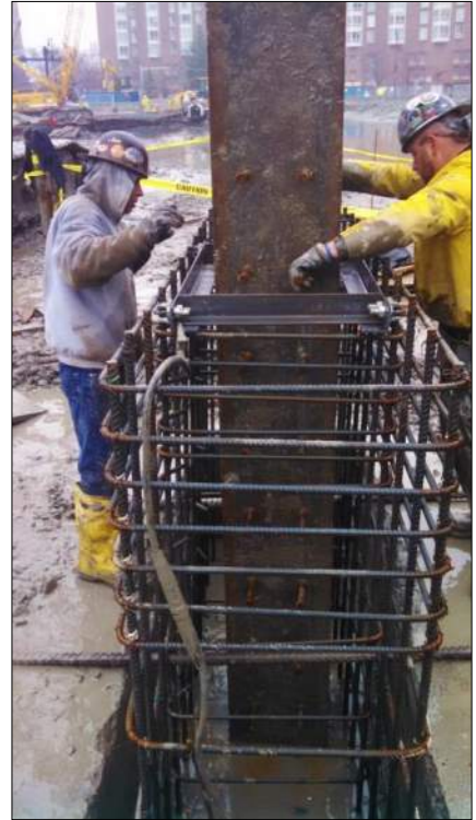
LBE Column Installation
