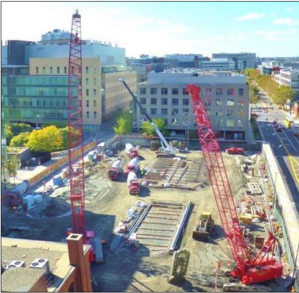
Slurry Wall Under Construction
