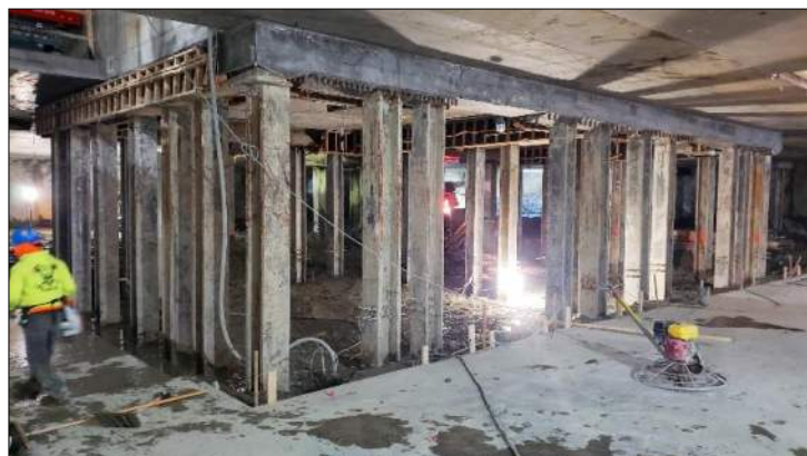
Exposed Columns at Basement Level 4
