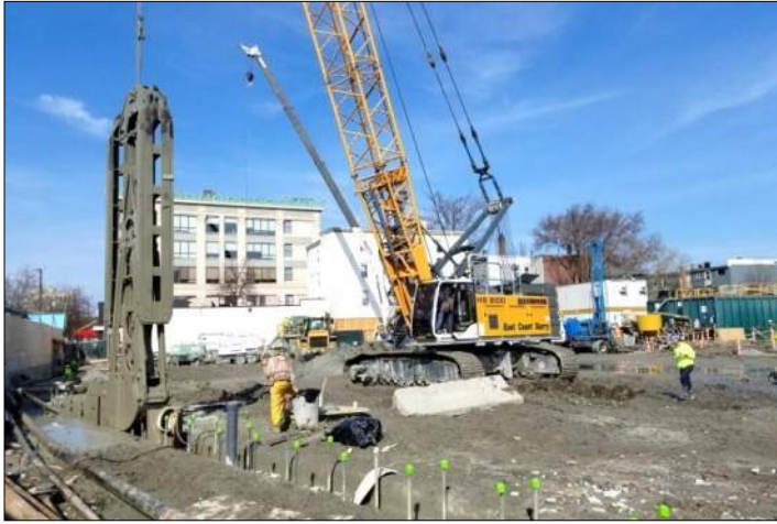
Panel Excavation Adjacent to Red Line Tunnel
