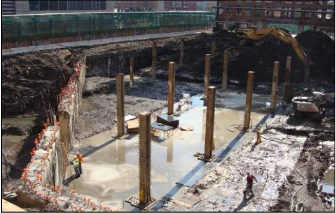
Exposed Slurry Wall and Top Down Columns
