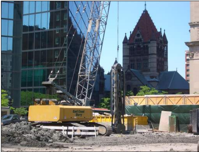
Slurry Wall Construction
