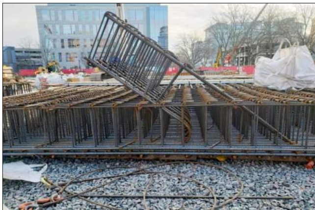
'Y' Panel Reinforcing Cage
