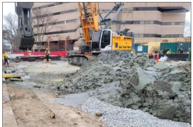
Slurry Wall Excavation in "WOR" Clay
