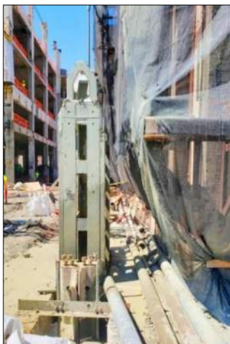
18" from Existing Building
