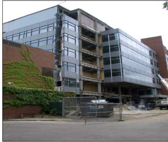
Superstructure Going Up
