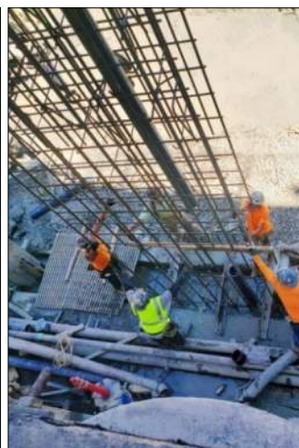
Cage Splice "Over the Hole"
