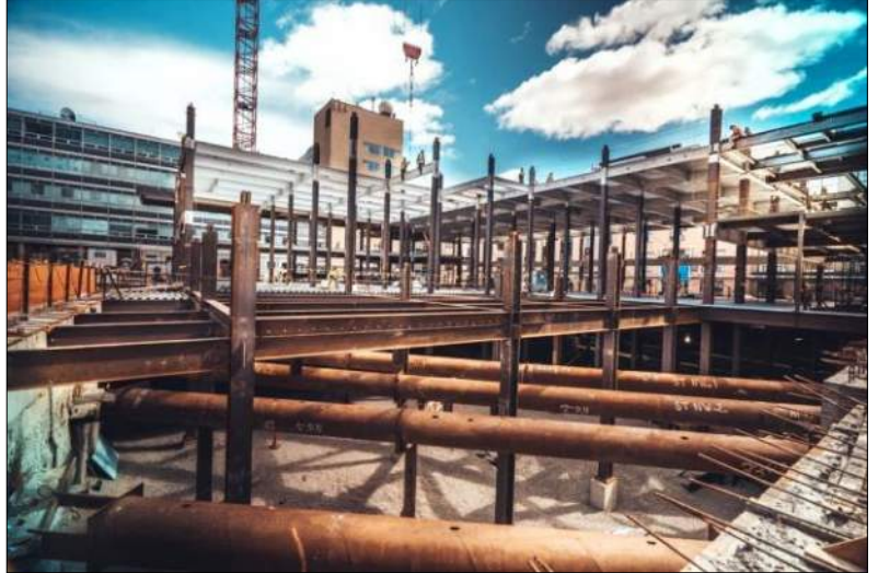
Building Frame Assembled through Bracing
