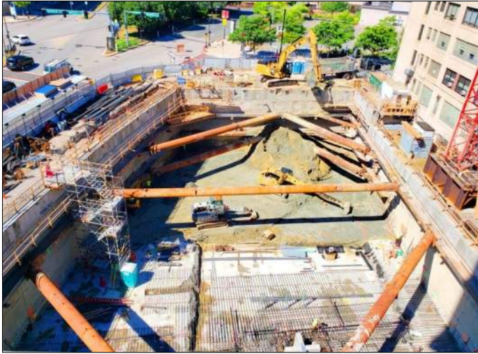
Completed Slurry Wall
