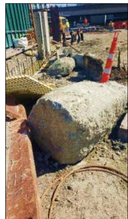
Various Obstructions Encountered During Slurry Wall Excavation
