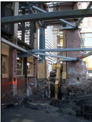
Pretrenching Underneath the Building Façade
