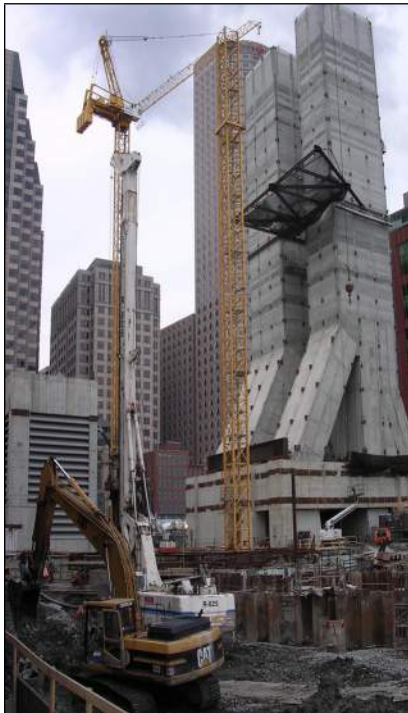
Drilling of Shaft Near Central Artery Vent Building
