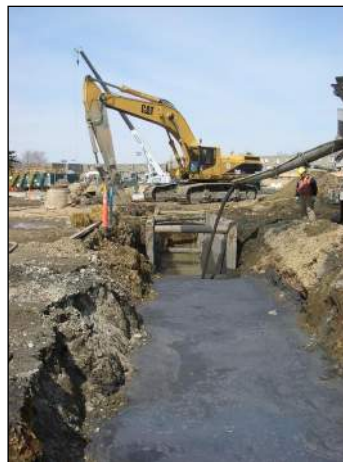
C-B Slurry Trench
