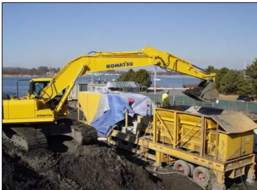
Backfill Mixing Plant
