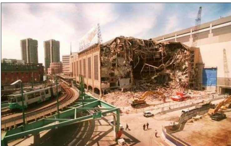
Original Garden Being Demolished in 1998
