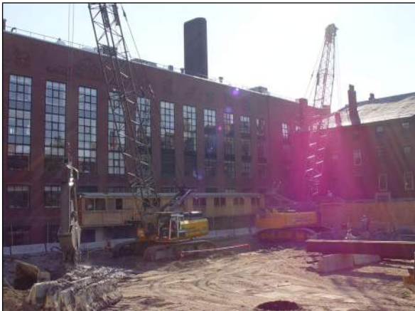
Slurry Wall Excavation in Progress
