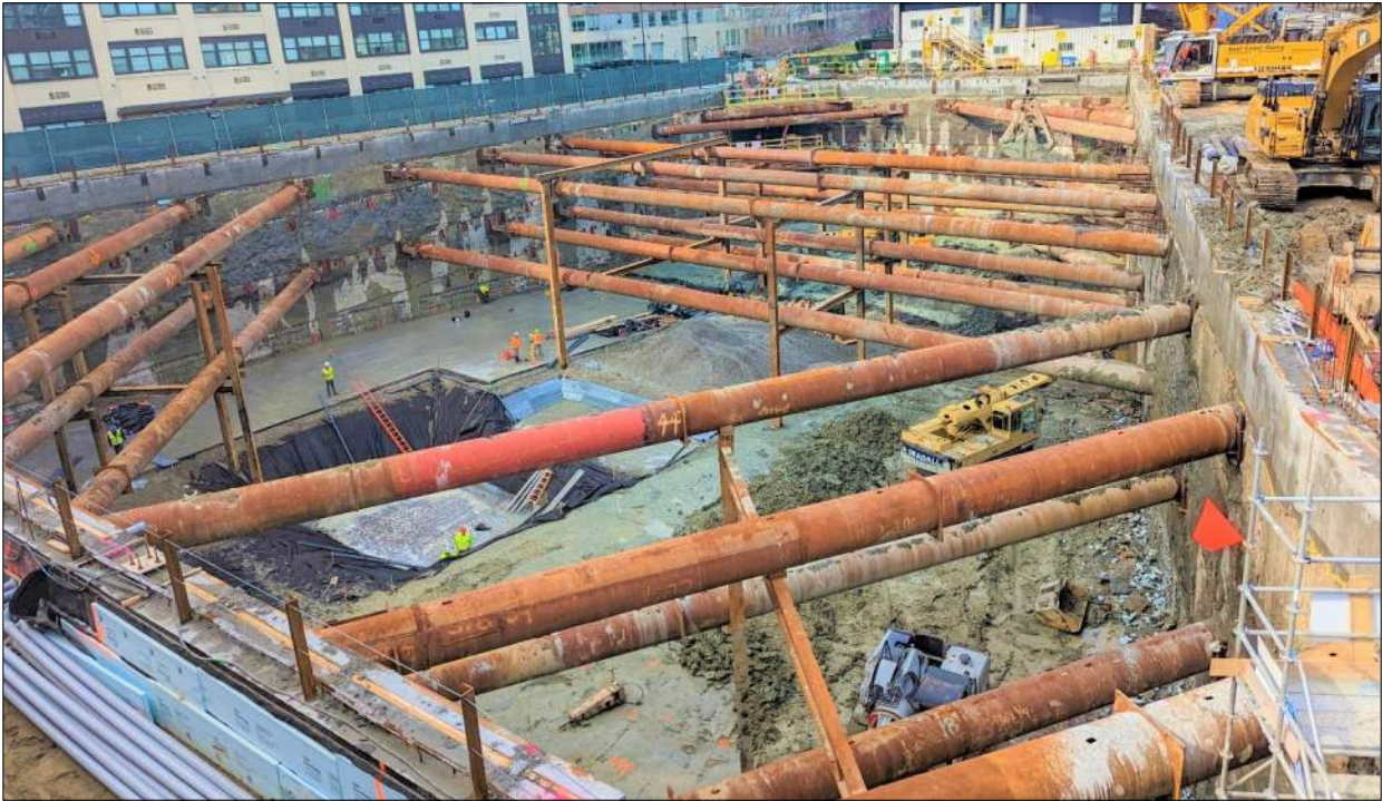
Exposed Slurry Wall Excavated to Subgrade
