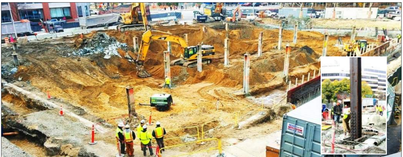
Excavation to B1 Level with Exposed LBE Columns
