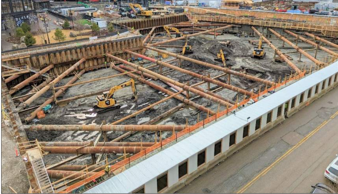
Permanent Slurry Wall on 2 Sides Braced to Temporary Sheeting
