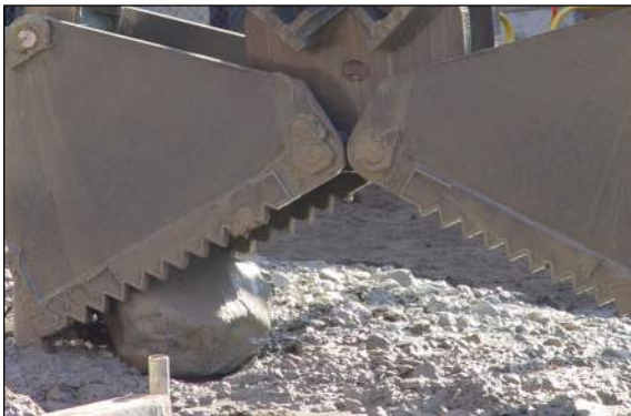
Clamshell Bucket Digging Glacial Till
