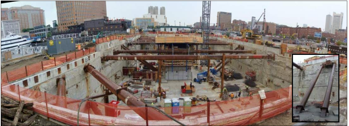
Mass Excavation Inside Braced Slurry Wall On Boston's Waterfront
