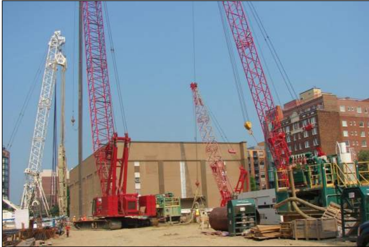
Three Clamshell Rigs and Hydromill
