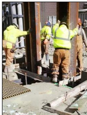
Core Wall LBE Columns Being Installed
