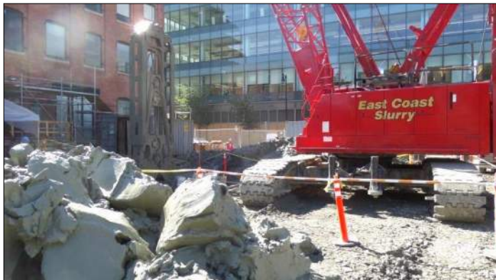
Clamshelling through Boston Blue Clay
