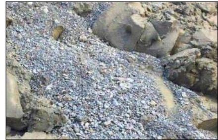
Slurry Wall Construction
