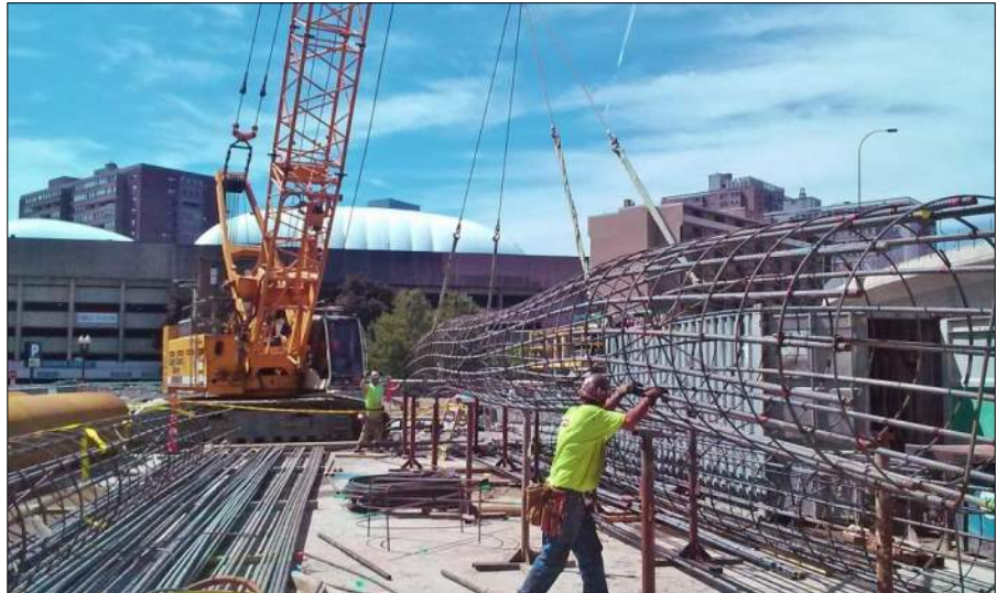
Shaft Reinforcing Cages
