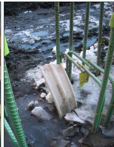
Installed Waterstop
