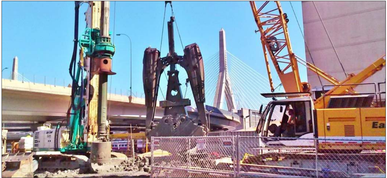
Drilled Shaft and LBE Construction
