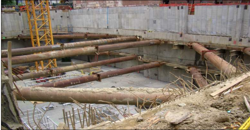
Braced Slurry Wall
