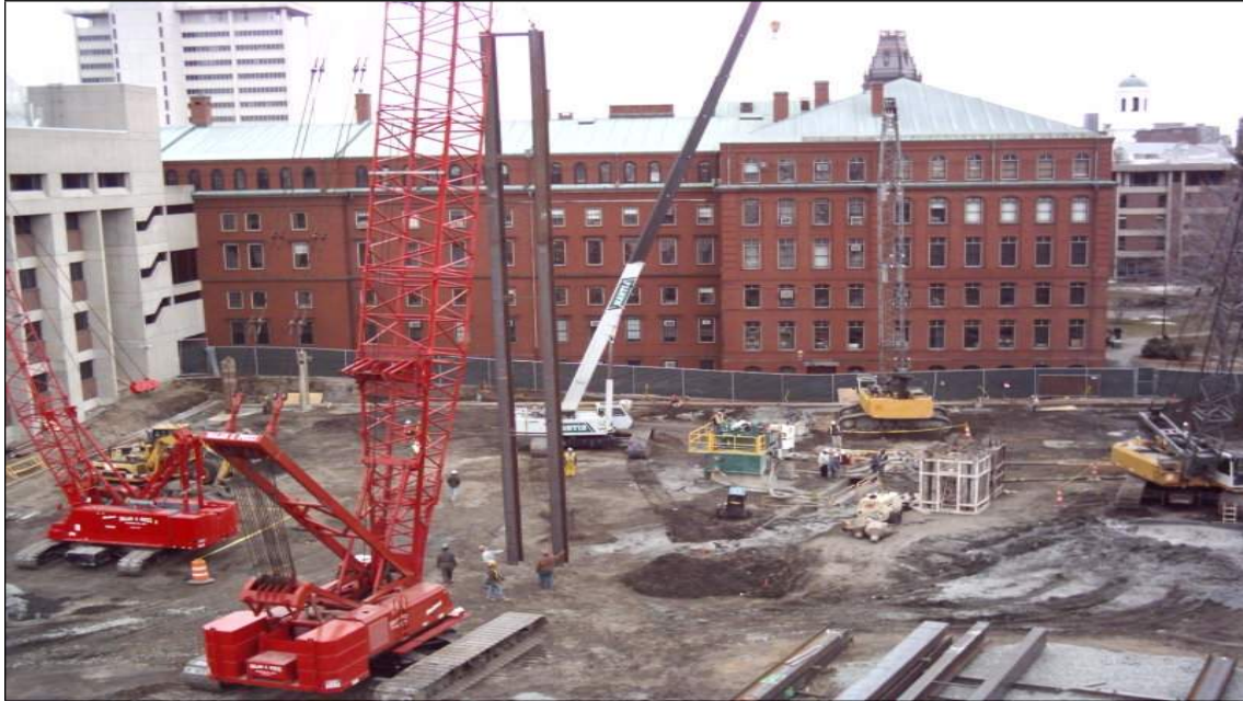
Placement of Soldier Piles Laced in Pairs
