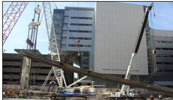
Heavily Reinforced Cage
