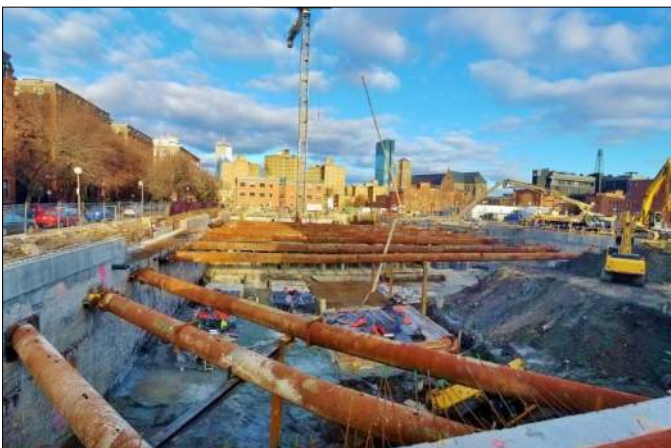
Braced Excavation
