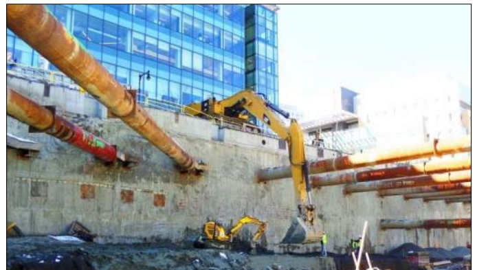
Completion of Bracing/Mass Excavation
