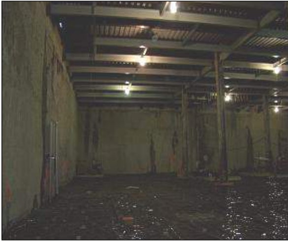
Basement Under Construction
