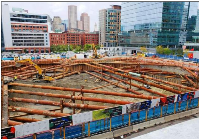
Three Levels of Bracing
