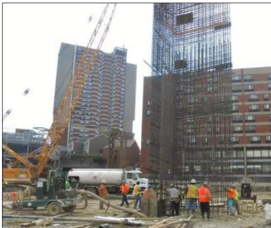
Reinforcing Steel Placement
