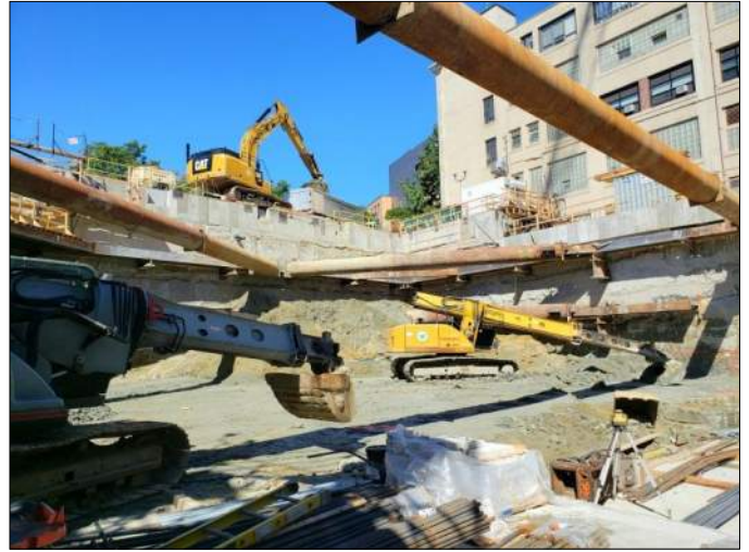
Completed Slurry Wall
