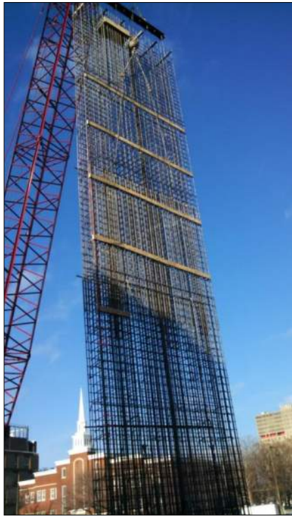
Wall Reinforcing Cage
