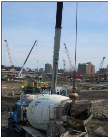
Wall Construction with 6 Cranes
