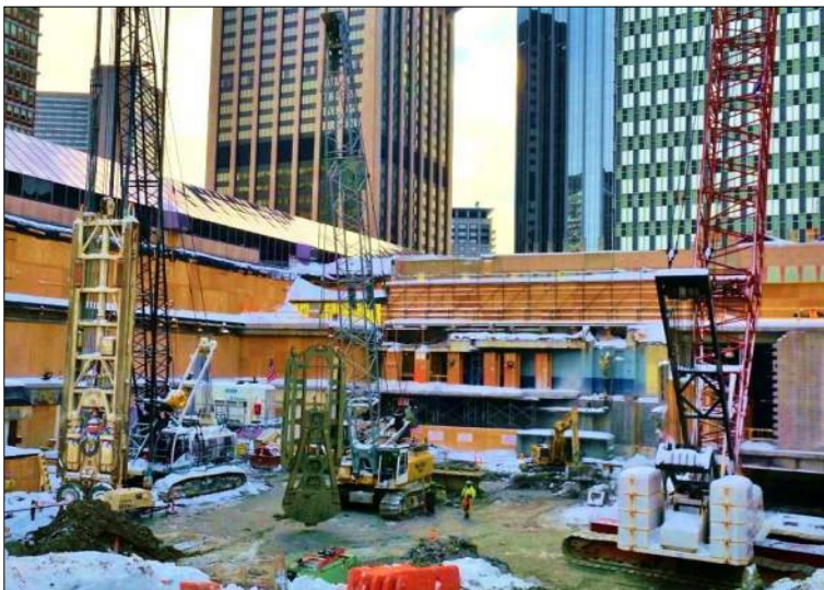
Excavation with Clamshell and Hydromill
