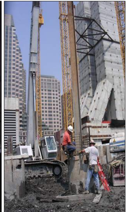
Placement of Embedded Column
