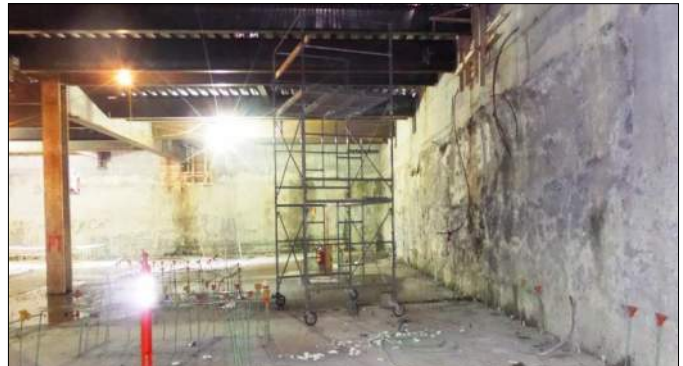
Exposed Slurry Wall and LBE Column
