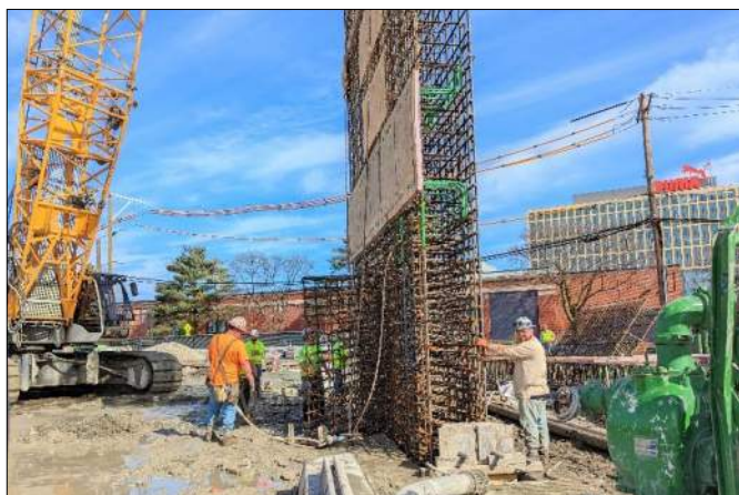
"Y" Panel Reinforcing Cage
