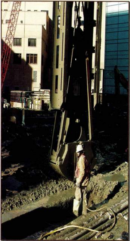
Twelve-ton bucket, wielded by Sennebogen Bauer crane, dwarfs worker as it is lowered into slurry trench.
