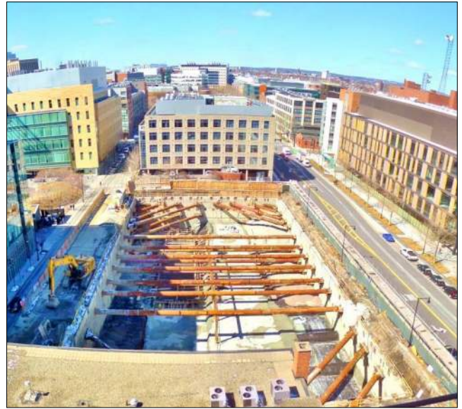
Braced Slurry Wall
