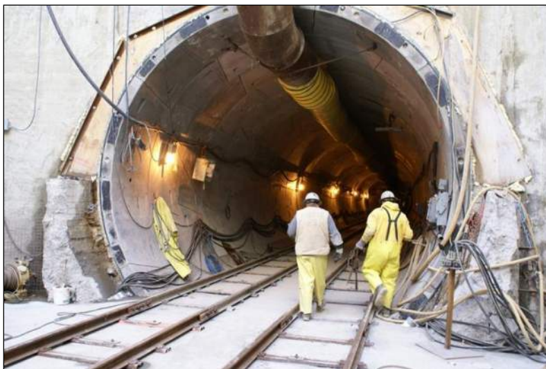
Tunnel Break Out at Access Shaft
