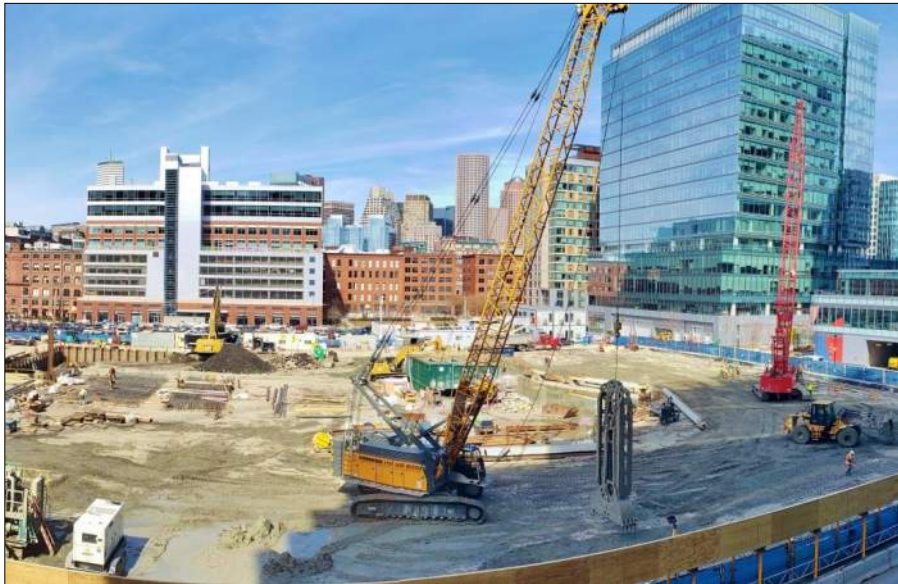
Slurry Wall Construction
