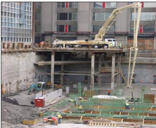
Wall & Shafts Support Concrete Pump
