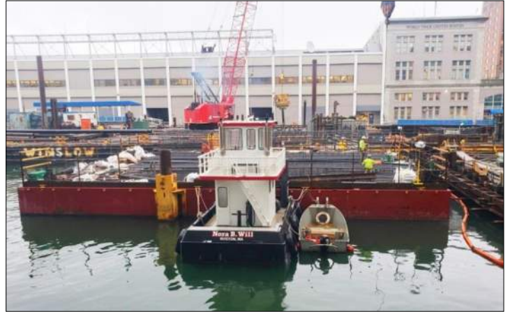
Barge Based Rebar Fabrication
