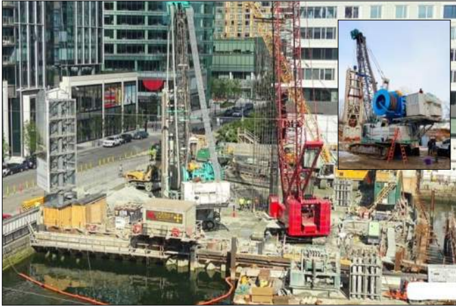
Slurry Wall Construction with Hydromill Rigged for 200' Depth (inset)
