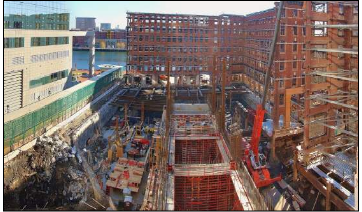
Top Down Construction Sequence
