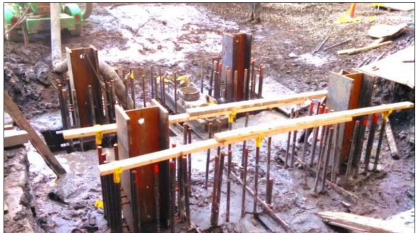
Tower Crane LBE Reinforcement
