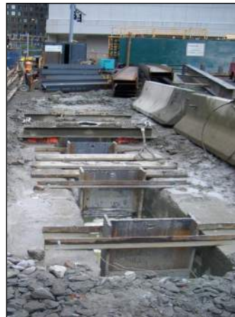
Installed Soldier Piles
