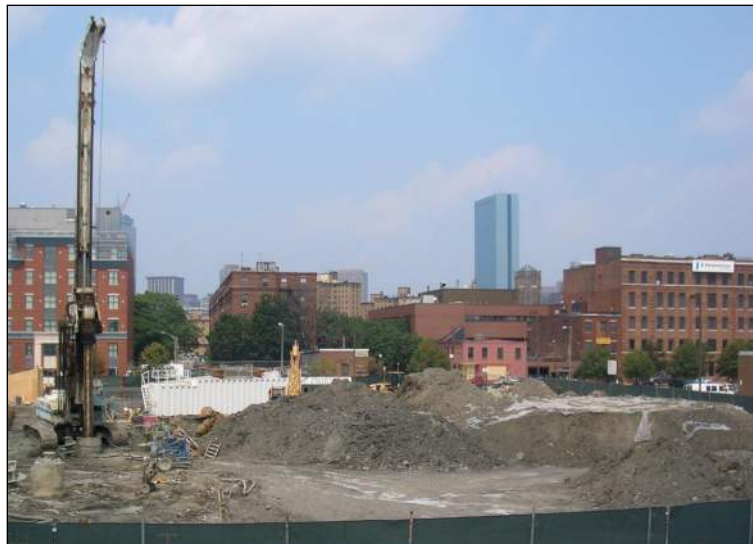
Stockpiled Drill Spoils for Disposal
