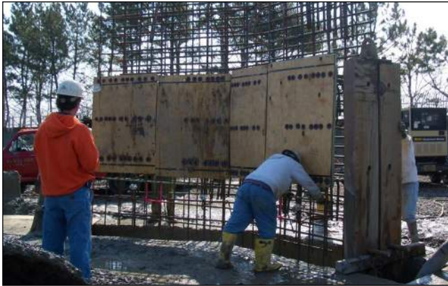
Main Access Shaft Slurry Wall Construction at Boston's Marine Terminal
