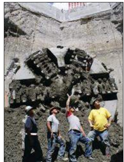
TBM Break In at Retrieval Shaft
