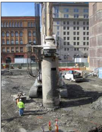
Coring thru Belled Caissons
