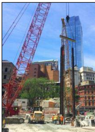
Core Wall LBE Columns Being Installed
