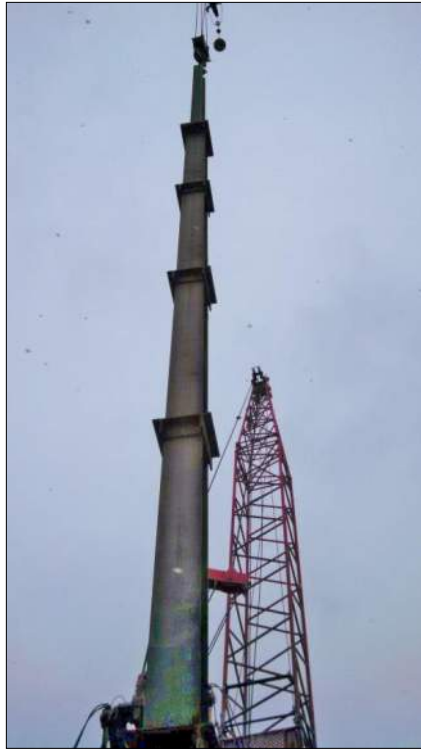
LBE Column Installation
