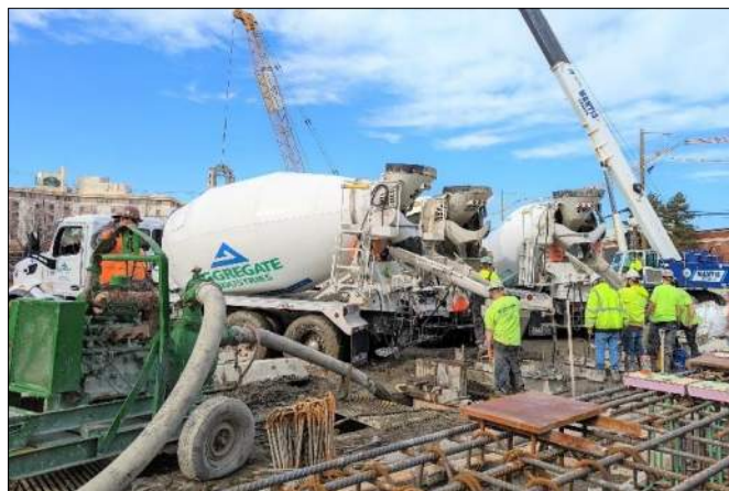
Tremie Concrete Placement
