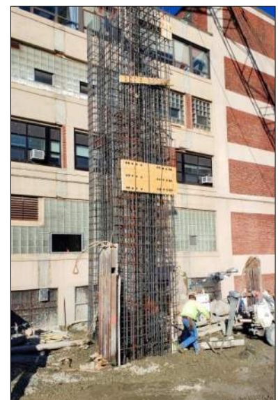
Reinforcing Cage Placement
