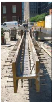
Column Shear Studs
