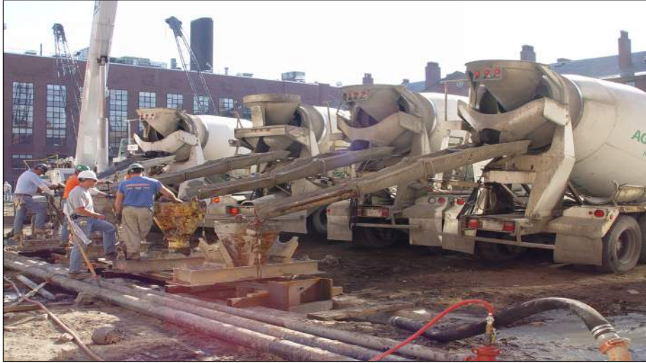
Tremie Concrete Placement
