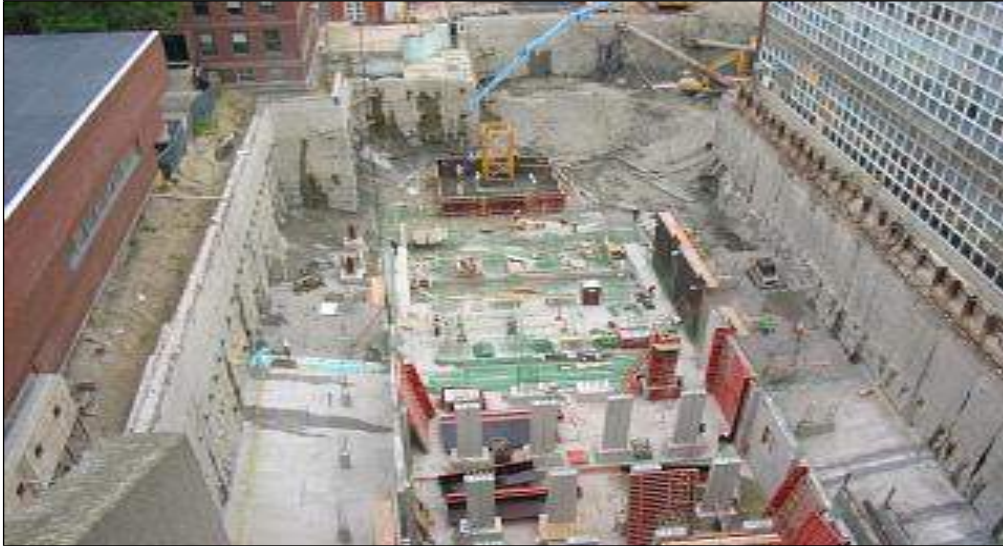
Slurry Wall Supports Adjacent Buildings
