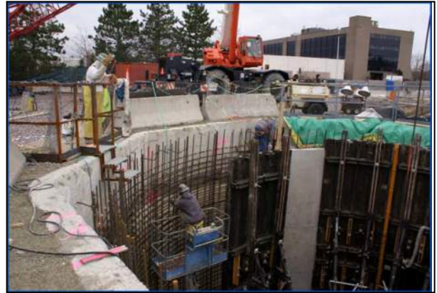
Main Access Shaft Slurry Wall Construction at Boston's Marine Terminal
