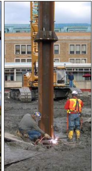
Column Connection to Reinforcing Cage
