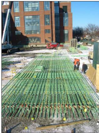
Epoxy Reinforcing Steel
