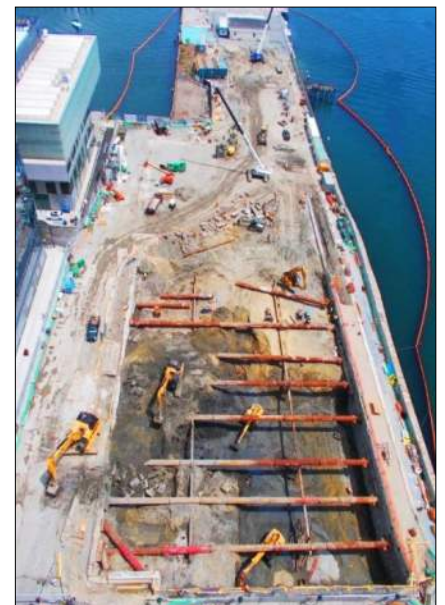
Start of Mass Excavation with Slurry Wall Still Under Construction
