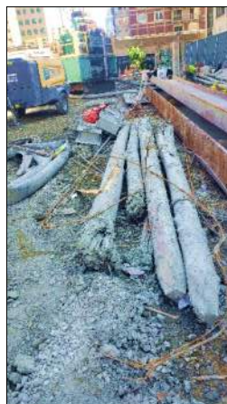
Various Obstructions Encountered During Slurry Wall Excavation
