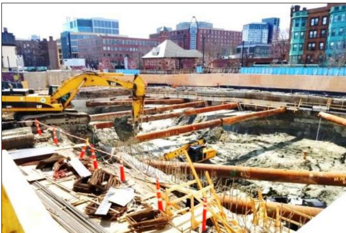
Braced Excavation
