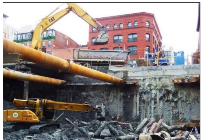
Exposed Slurry Wall with Remnants of Timber Piles from Original Garden
