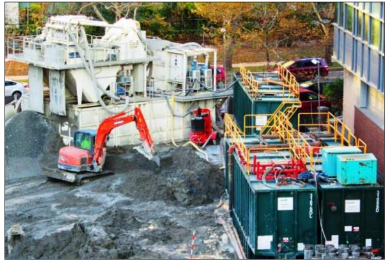
Hydromill Sotress Plant
