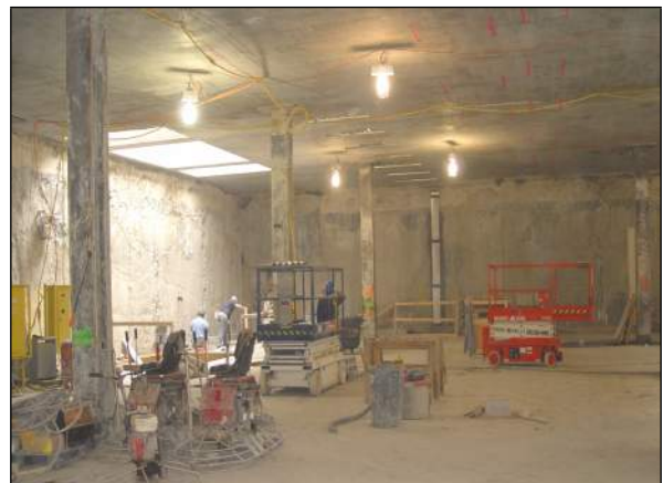
Exposed Wall and LBE Columns
