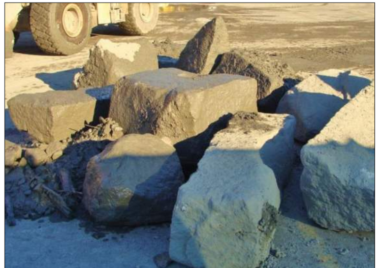
Seawall Blocks Removed During Slurry Wall Excavation
