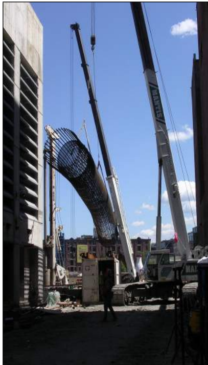
Placement of Shaft Reinforcement
