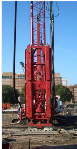
Mill Cutting Rock for LBEs
