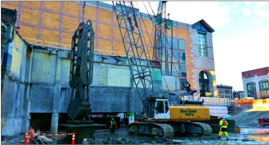
Clamshelling Overburden Soils
