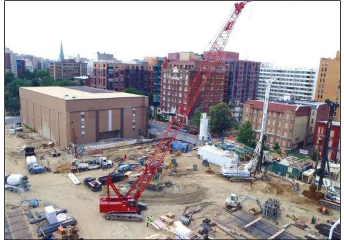
Drilled Shaft Construction
