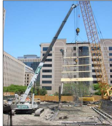
Reinforcing Cage with "Legs"
