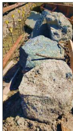
Various Obstructions Encountered During Slurry Wall Excavation
