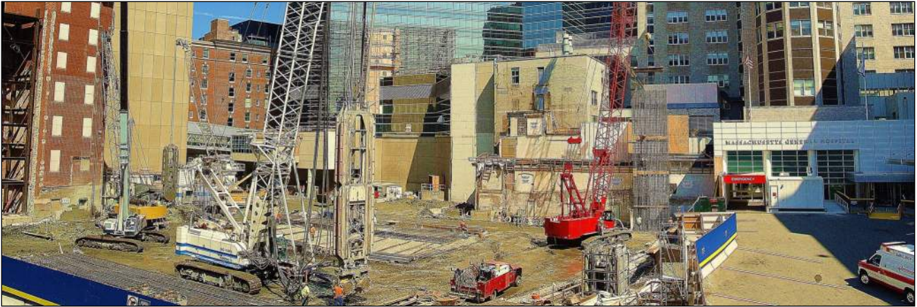
Wall Construction with Two Clamshell Rigs and a Hydromill
